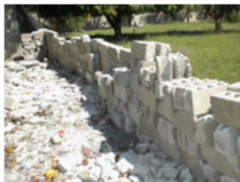
The damaged boundary wall
