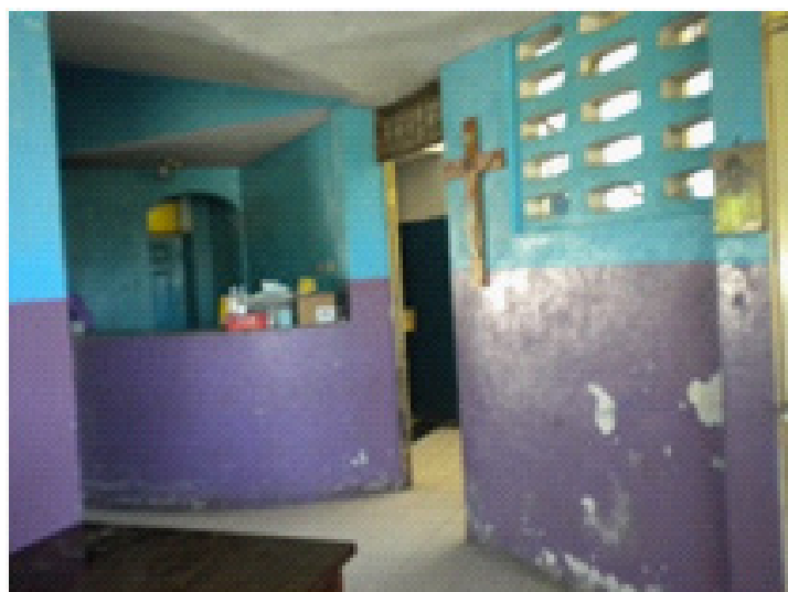
The damaged entrance to the Holy Angels Hospice in Haiti
